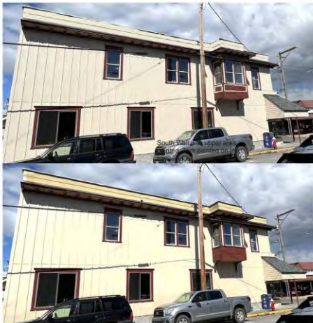
South Wall with upper area painted. Trim painted on the bay window.
