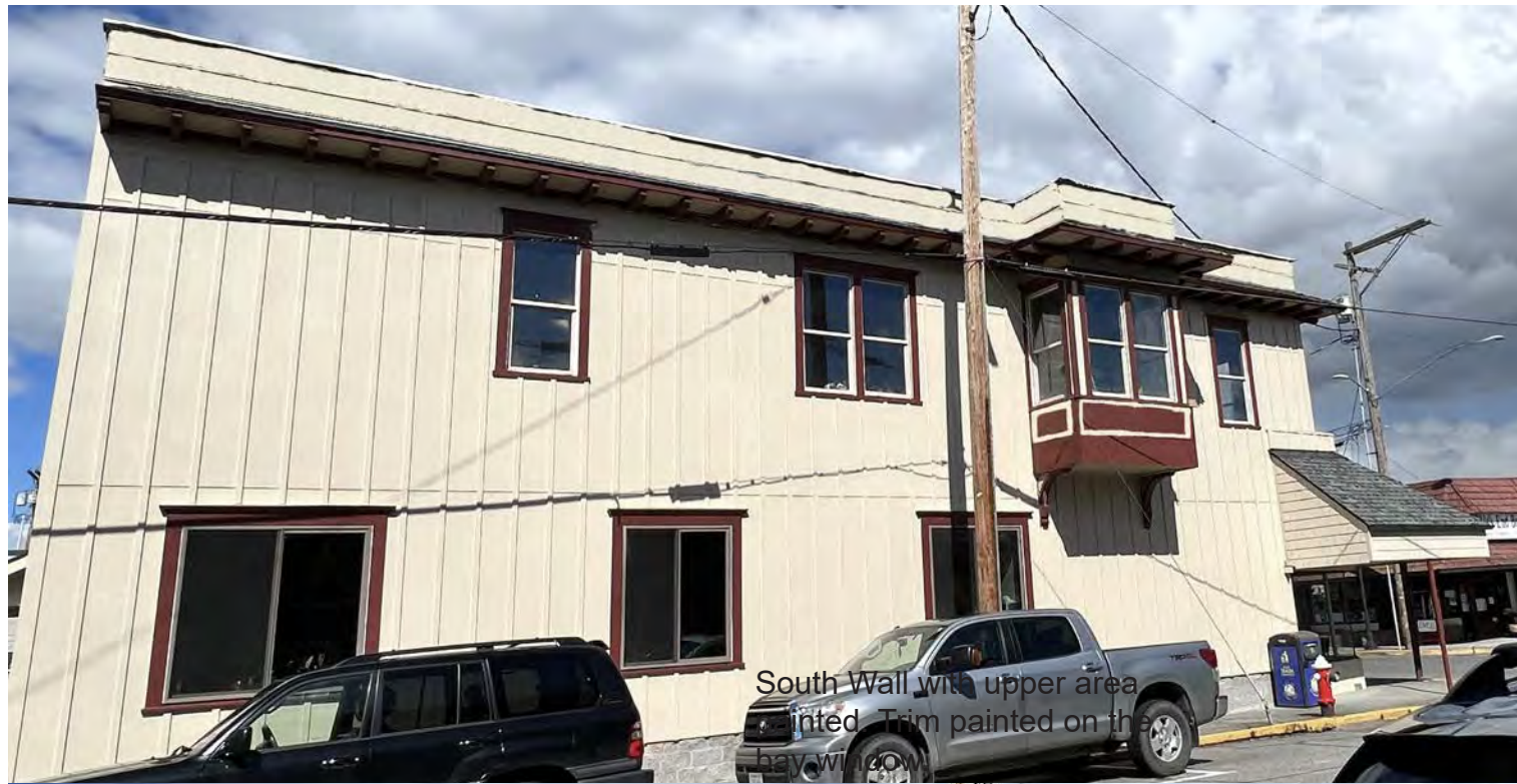
South Wall with upper area painted. Trim painted on the bay window.
