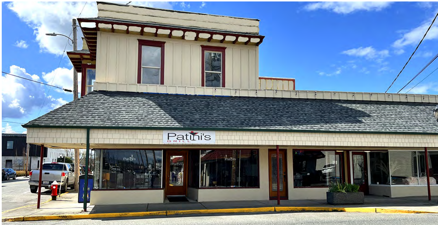
Front, east facing, painted.
