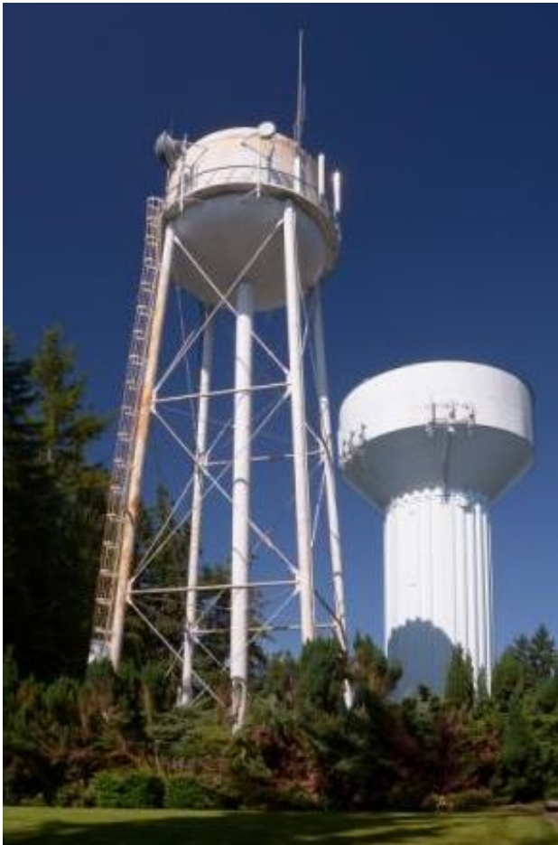
Lakewood, WA Water tanks #2, #3
