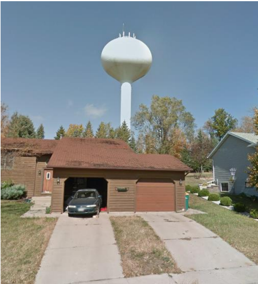
DISH WATER TOWER Installation #2, Rochester, Minnesota
