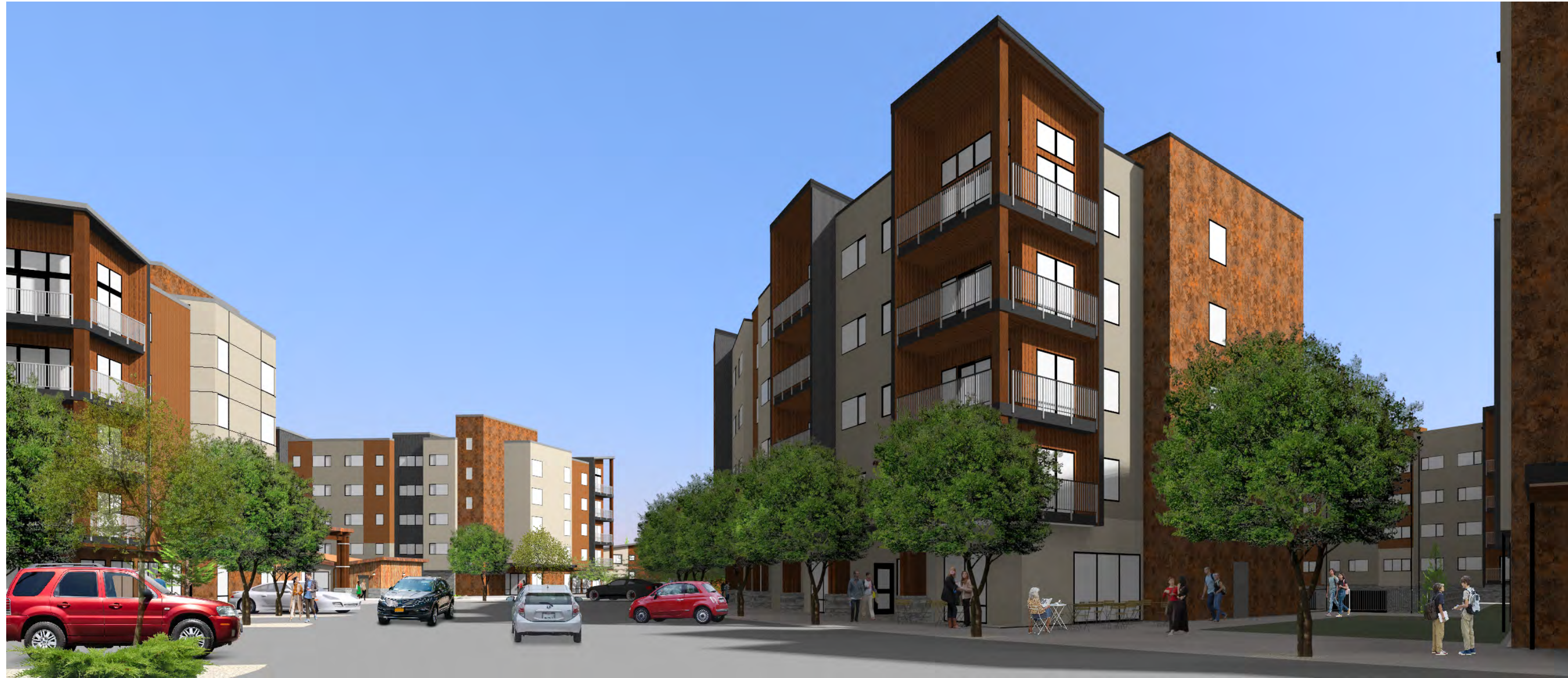
Mixed-Use Retail Looking East
