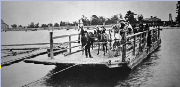
Camano Ferry, Photo provided by City of Stanwood
