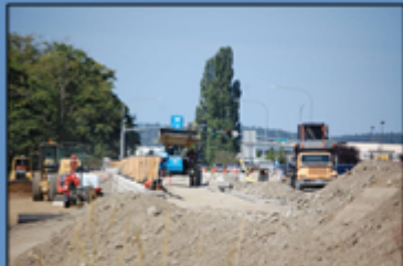
Construction work along Viking Way and 90th Avenue. Source: GoSkagit.com
