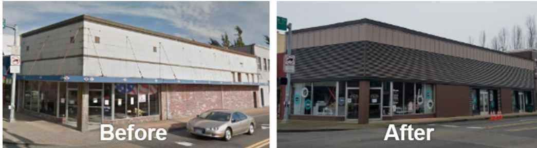
Auburn, WA Façade Improvement Grant Program – Painted lower story brick, added two doorways on west facing façade, removed awning, re-cladded upper story, and retained cornice
