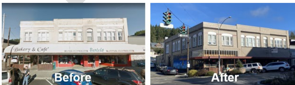
Chehalis, WA Façade Improvement Program
