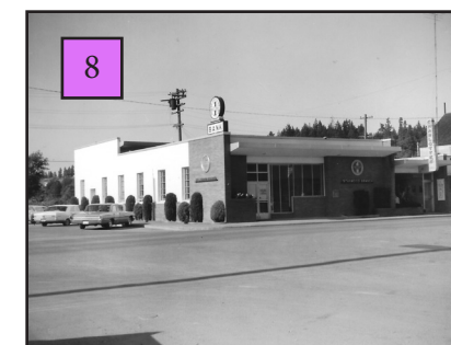
8 First National Bank (Police station)
