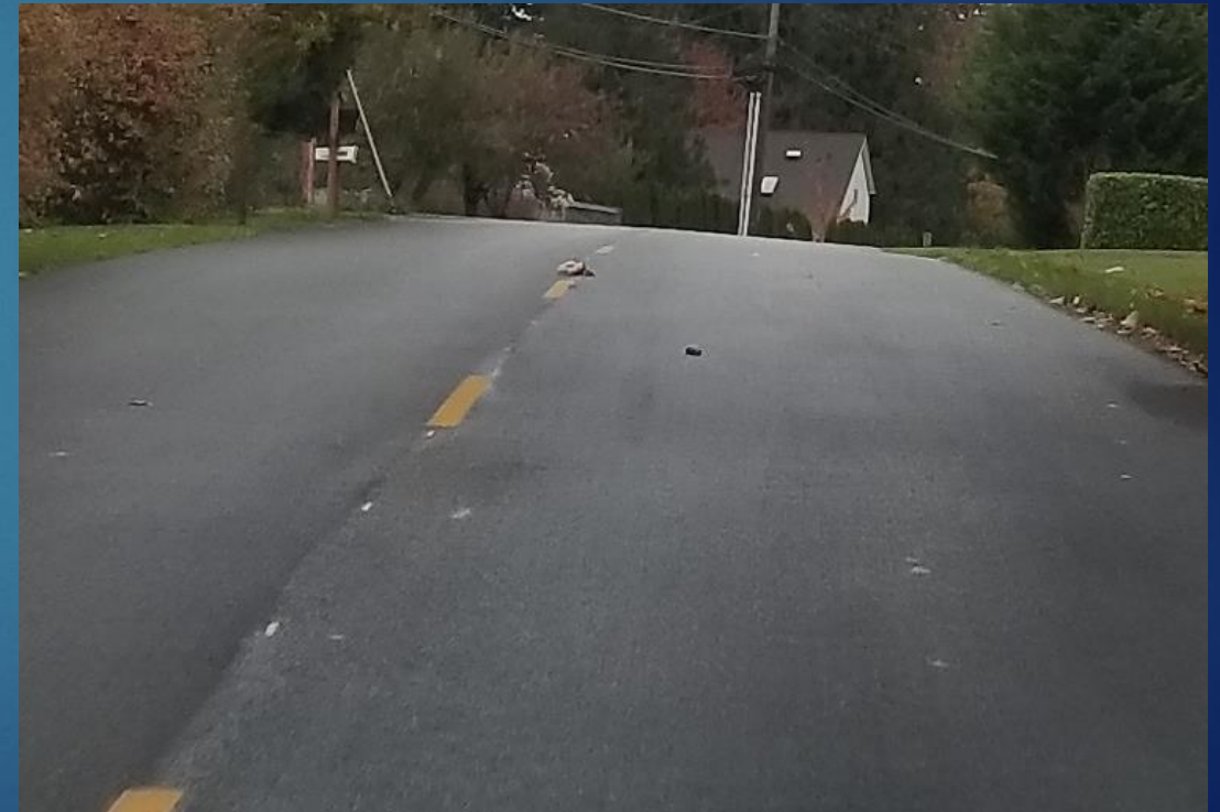
Looking northeast and up the hill on Cedarhome Drive
