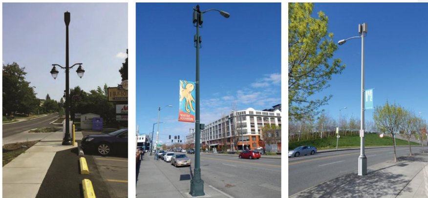
Examples of a well-designed small cell facility
