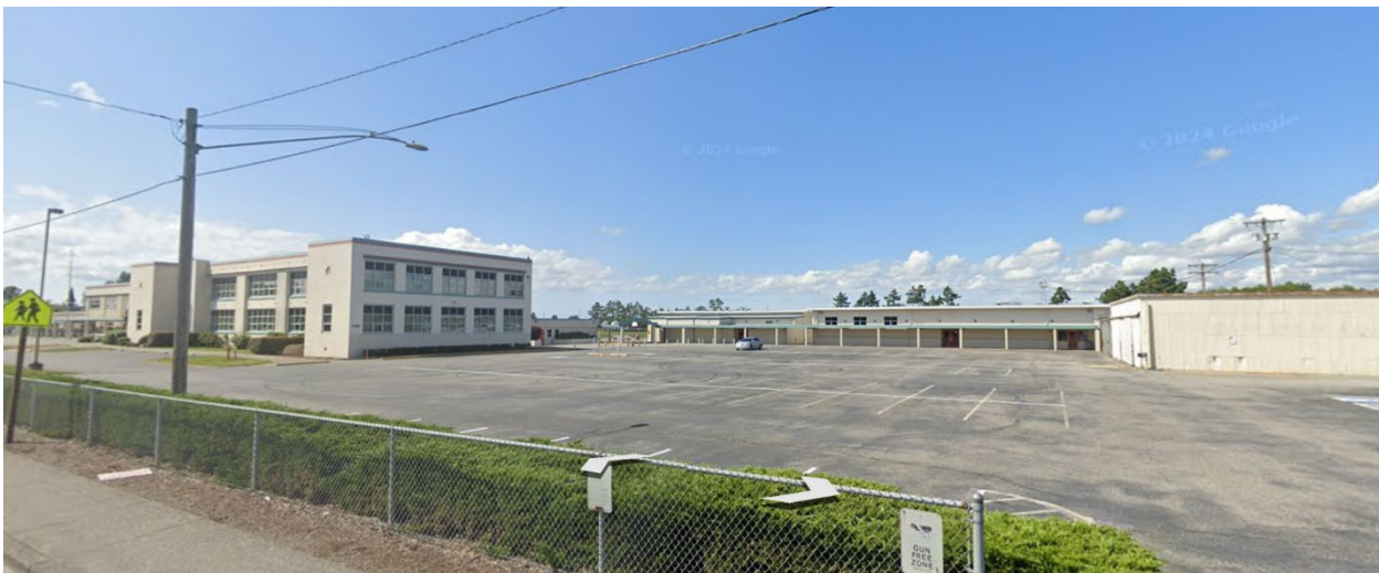
Stanwood Middle School - 9405 271st St NW
