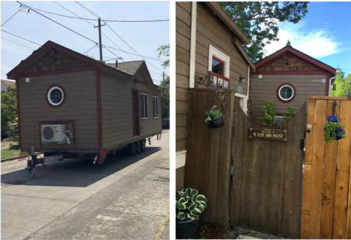
Prefab ADU travelling from factory to residential site / installed on-site. Credit: Roger Fitzsimons.
