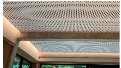
Ceiling installed acoustic panels in a common area. Photo courtesy of Schemata Workshop.
