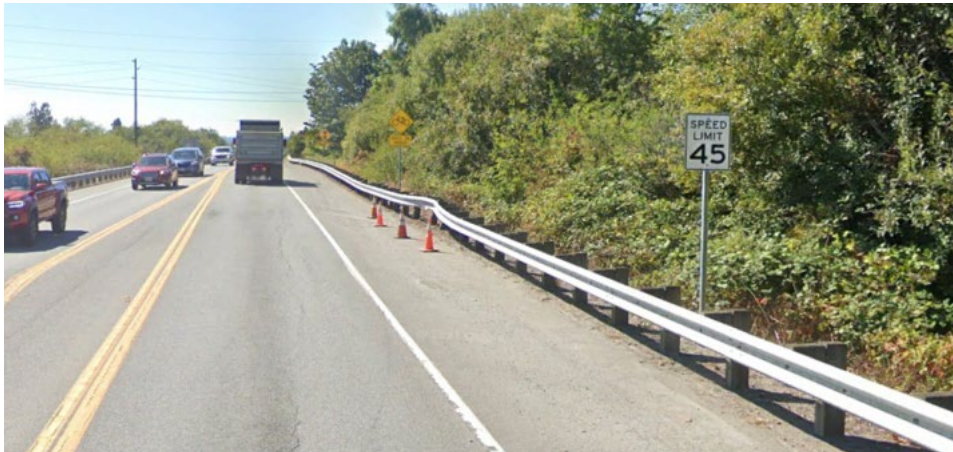
45 mph Speed Limit on SR 532 Between Pioneer Highway and 88 th Avenue
