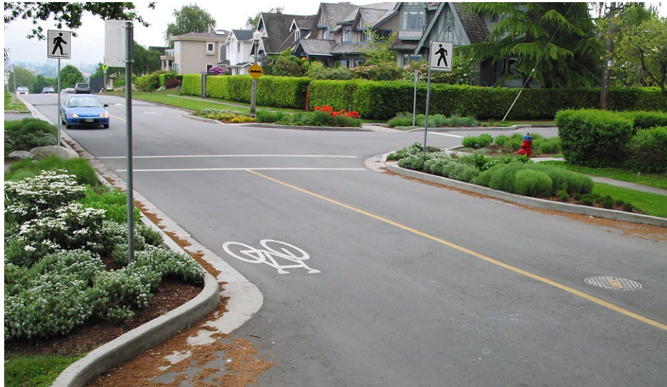
Figure 11.12.010(C) Bump-out Crossing Example (Credit: Richard Drdul)
