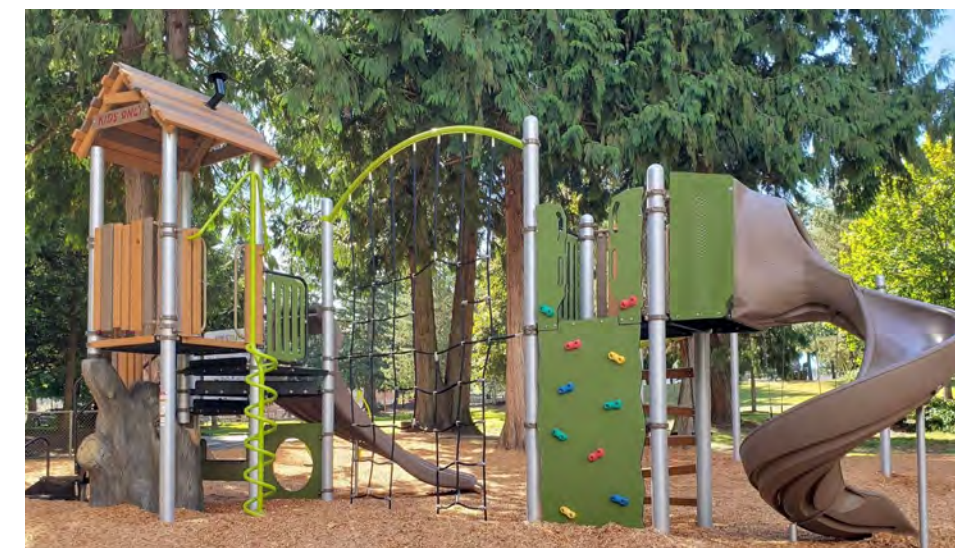
Image: The Church Creek Park playground was recently updated with new play equipment.
