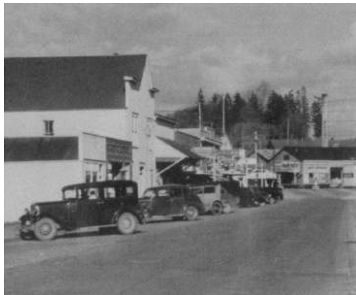
East Stanwood, Photo provided by City of Stanwood
